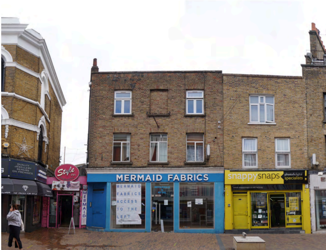
Fig 2. Existing Street Frontage
